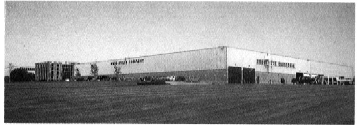
Webb-Stiles Company, main plant and corporate offices in Valley City, Ohio.
