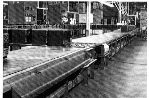
Steel slat conveyors being used in a major appliance manufacturing plant. The ball top table transfers built along the line allows transfer of appliances to inspection loops.
