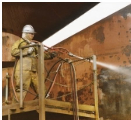
High Pressure Wet-Blasting System
