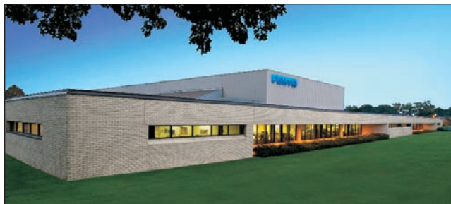
East: 395 Moreland Road, Hauppauge, NY 11788
