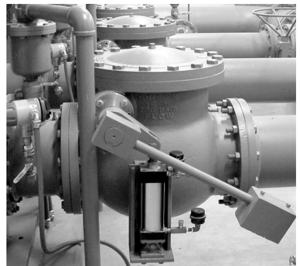
12" air-cushioned Swing Checks are shown at a recent Crispin installation. The air valves in the photo are also from Crispin.
