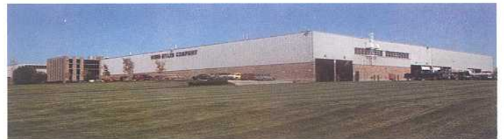
Webb-Stiles Company, main plant and corporate offices in Valley City, Ohio.
