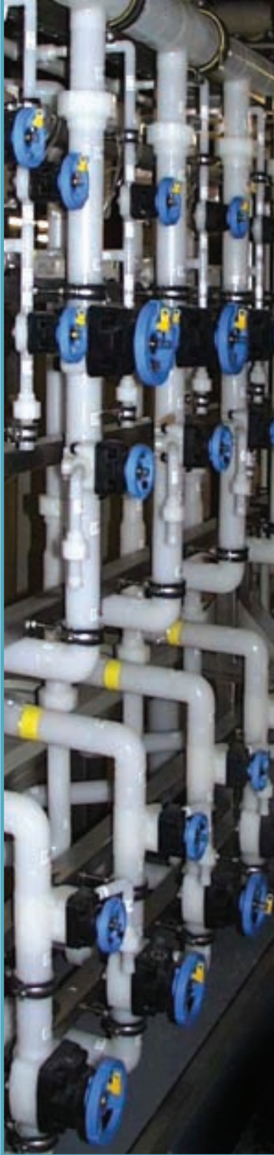
A high purity application of Purad pipe, valves, and fittings.
