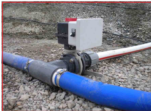
QM Remote Cycle™ w/Series 94 Actuator & Type-57 Butterfly Valve
