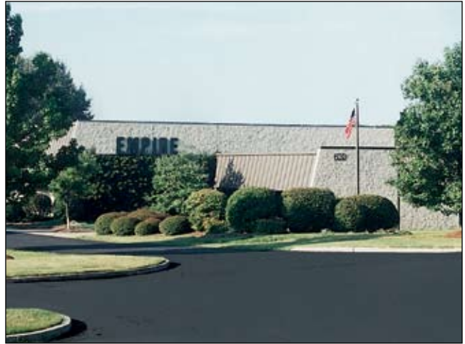
Empire Abrasive Equipment Company, headquartered in Langhorne, Pennsylvania, specializes in the development of air-blast systems and equipment.
